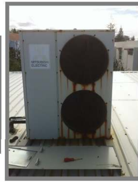
Actual instances of case corrosion which could have been prevented with a CAT
