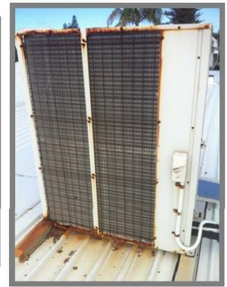
Actual instances of case corrosion which could have been prevented with a CAT
